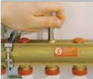
LOCKSHIELD VALVE OPENING
